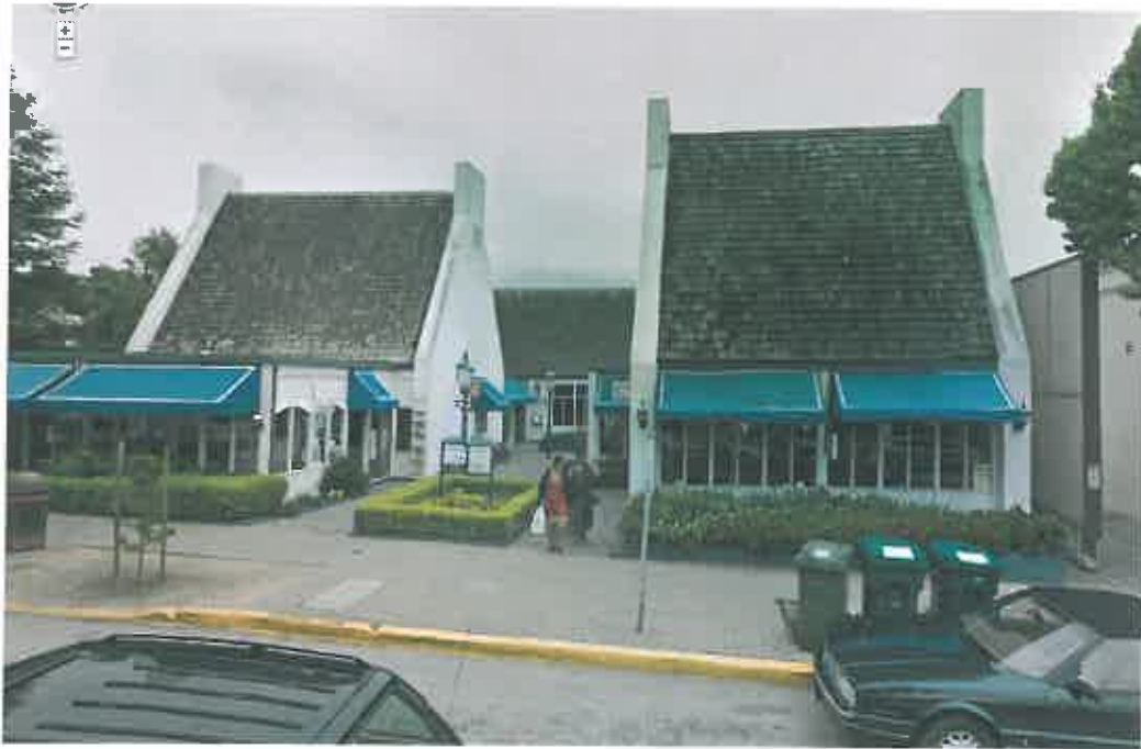
Carmel Square Courtyard facing east – Project site located at rear of courtyard
