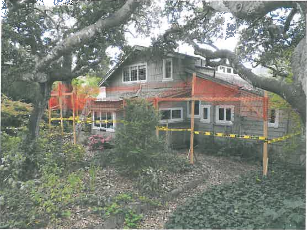
Rear of residence, area of addition
