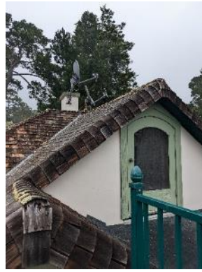
Sunroom roof to be repaired; carpeting will be removed, water barrier reinforced; proper surface installed; and railing affixed.
