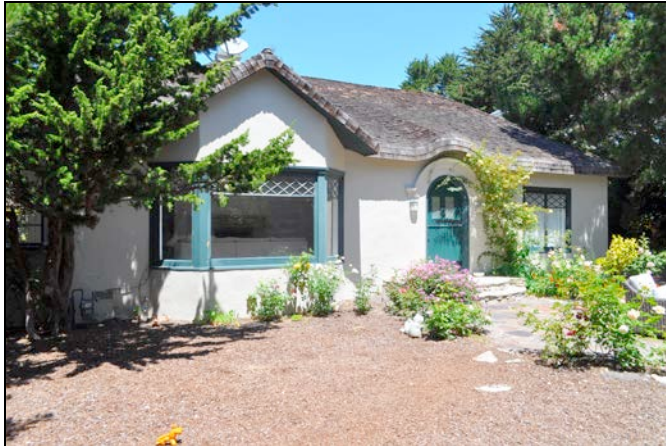
Figure 1. Front (east) elevation.
