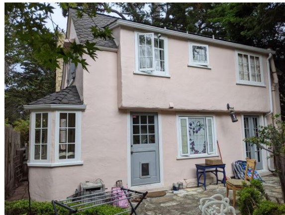
Rear (east elevation), looking northwest.
