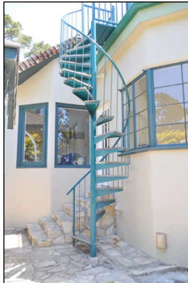
Figure 4. Metal spiral staircase.
