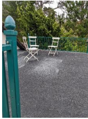
Sunroom roof to be repaired; carpeting will be removed, water barrier reinforced; proper surface installed; and railing affixed.
