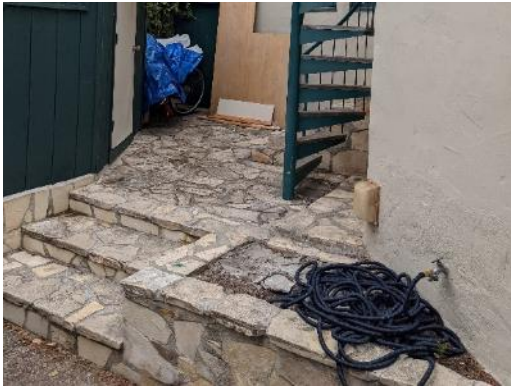
Broken landing and step stonework will be repaired.
