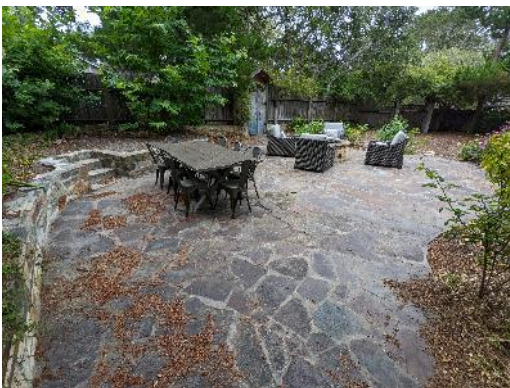
Patio stonework will be regraded to direct water away from the home.
