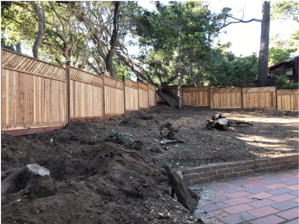
Figure 1 View of removed trees - stumps under hand ex
