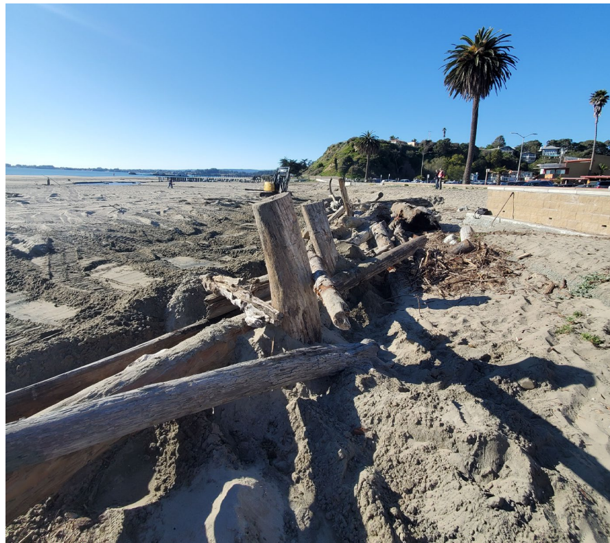
Living Shoreline Construction in Aptos
