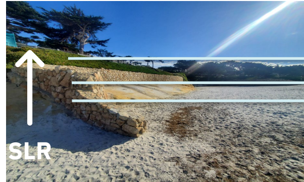
The light blue lines indicate the higher water level exposure with sea level rise
