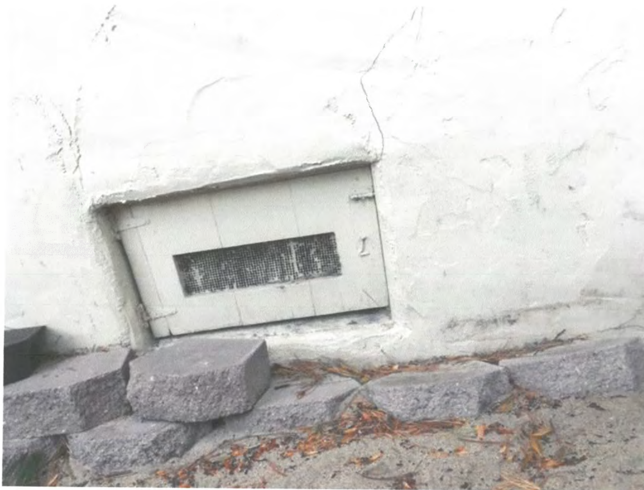
Foundation vent 5, crawl space door
