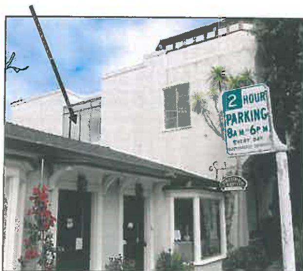
Figure 5. View of south elevation, with an arrow showing the non-historic glass screen blocking original lightwell.
