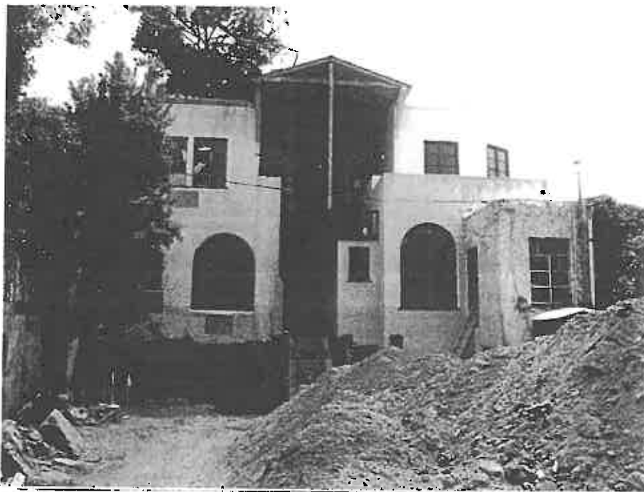
Looking east at the rear (west) elevation, 2014.
