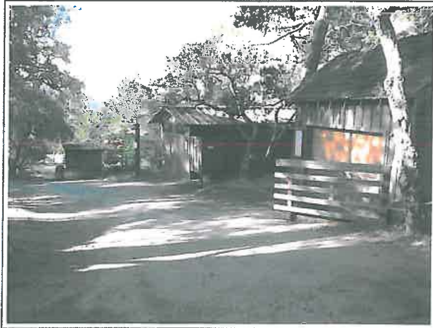
Photograph 8. Concession building (right), restrooms (center) and ticket booth.
