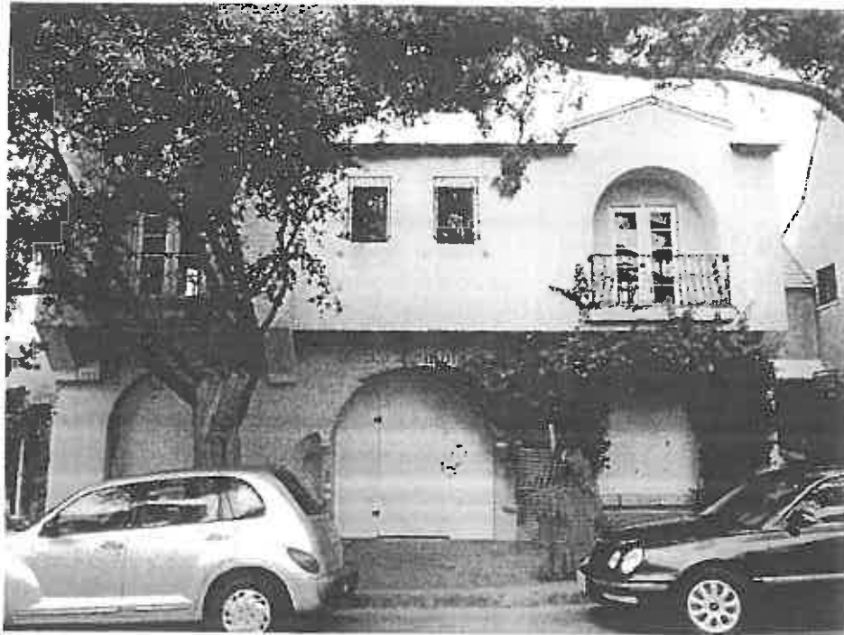
Looking west at the east facing facade, 2014.
