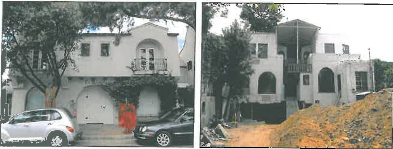
Figures 1 and 2. Left image shows the La Rambla Building's front (east) elevation. Existing historic wrought iron window surrounds and balcony railings will be restored. Right image shows the rear (west) elevation. The existing historic wood bridge and railings between the upstairs apartments will be retained and restored.
