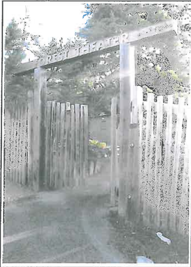
Photograph 12. Pedestrian entrance along Santa Rita Street.
