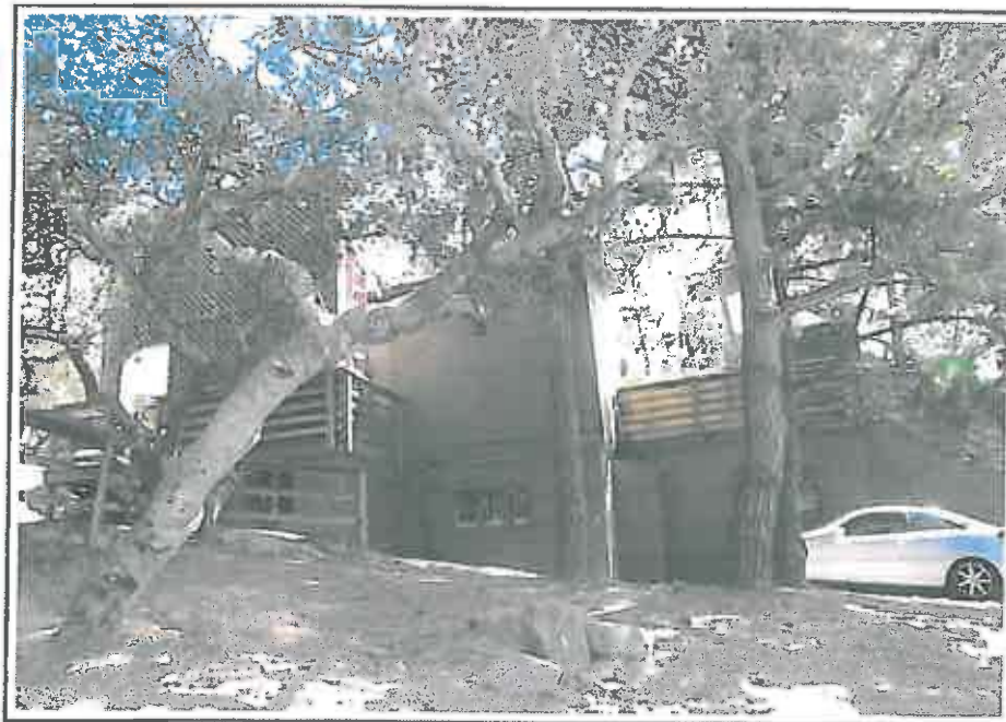
Photograph 3. West side of stage.
