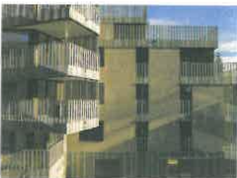
oko skin 147 mm, various colours, vertical installation, rivets on aluminium substructure
