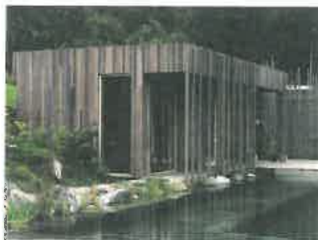
oko skin flex 125 mm, various colours, vertical installation, rivets on aluminium substructure
