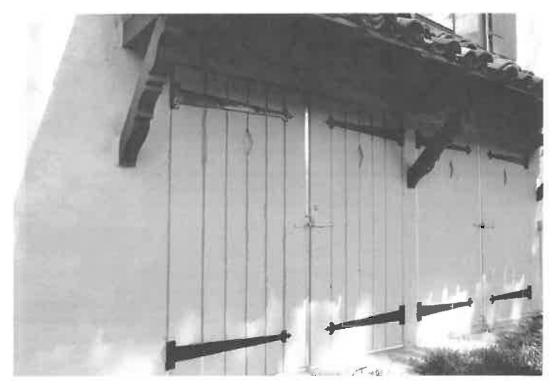
Photo #3. Looking at the south facing garage doors that are backed with plywood, & painted to appear as vertically planked wood, Kent Seavey, 4/3/2017.
