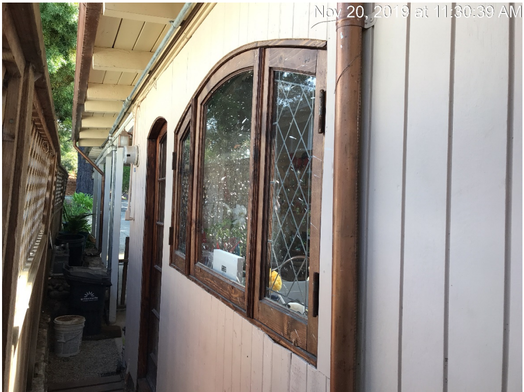
Fenestration not original to residence
