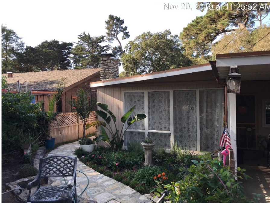
Front elevation fenestration is original and intact with two "sun sash" (jalousie) windows under fixed pane windows (left side)
