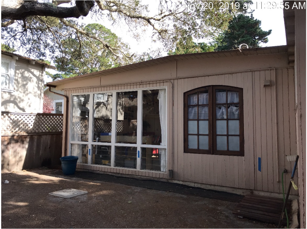
Rear Elevation: Left side fenestration original and intact; Right side fenestration has been modified
