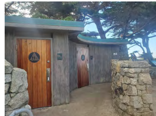
Restroom near Santa Lucia Ave
