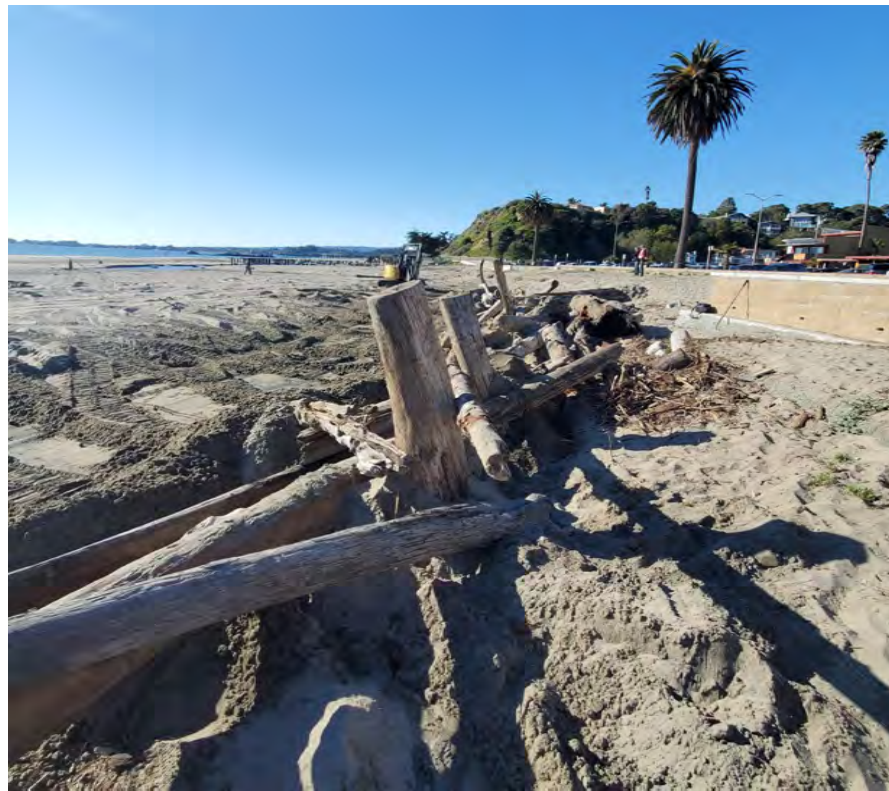
Living Shoreline Construction in Aptos
