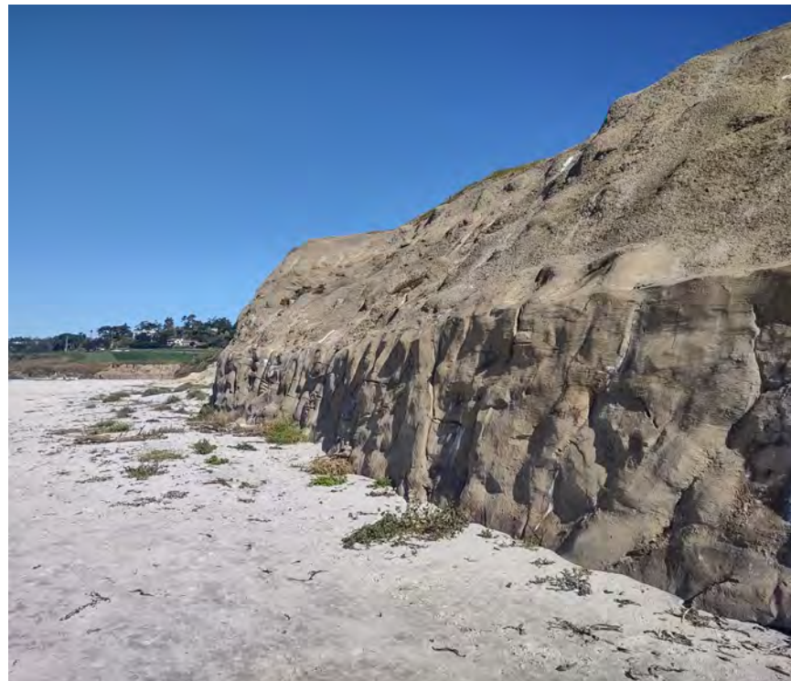
Shotcrete wall at Pebble Beach Golf Links
