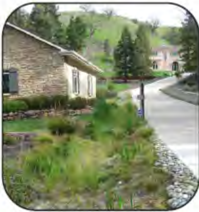
Large Residential Rain Garden
