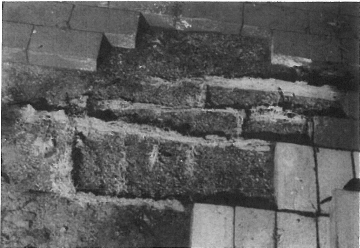
Figure 11. Roots growing in the crevices between bricks. There was no oxygen below the bricks that overlaid a compacted clay soil on the North Carolina State University campus. Tree roots commonly follow cracks, crevices, and other air passages underneath pavement. Photo by T. O. Perry.
