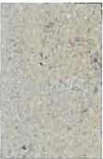
Example Of Concrete Walk
