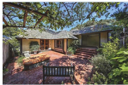
EXISTING PATIO / ENTRY (EAST)
