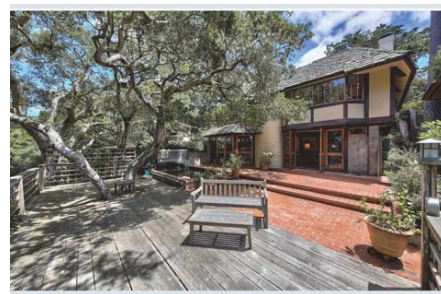
EXISTING REAR (WEST) FACADE
