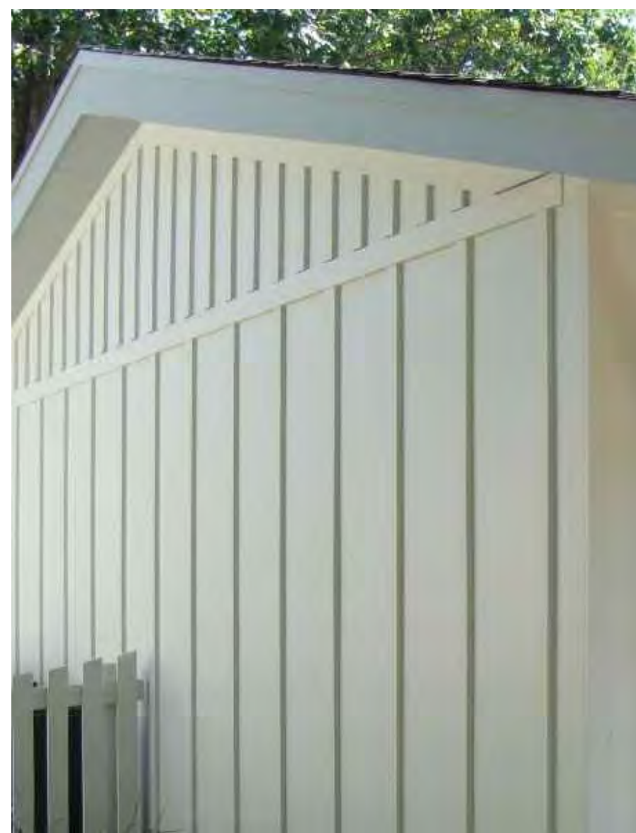
4 PAINTED WOOD. BOARD & BATTEN SIDING COLOR: WHITE
