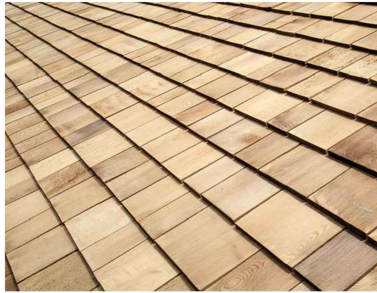
1 CLASS 'A' WOOD CEDAR SHAKE ROOF
