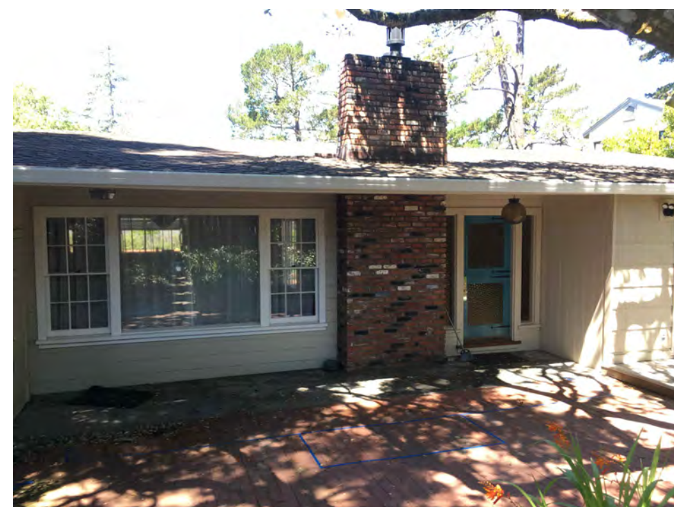
FRONT ELEVATION LOOKING WEST
