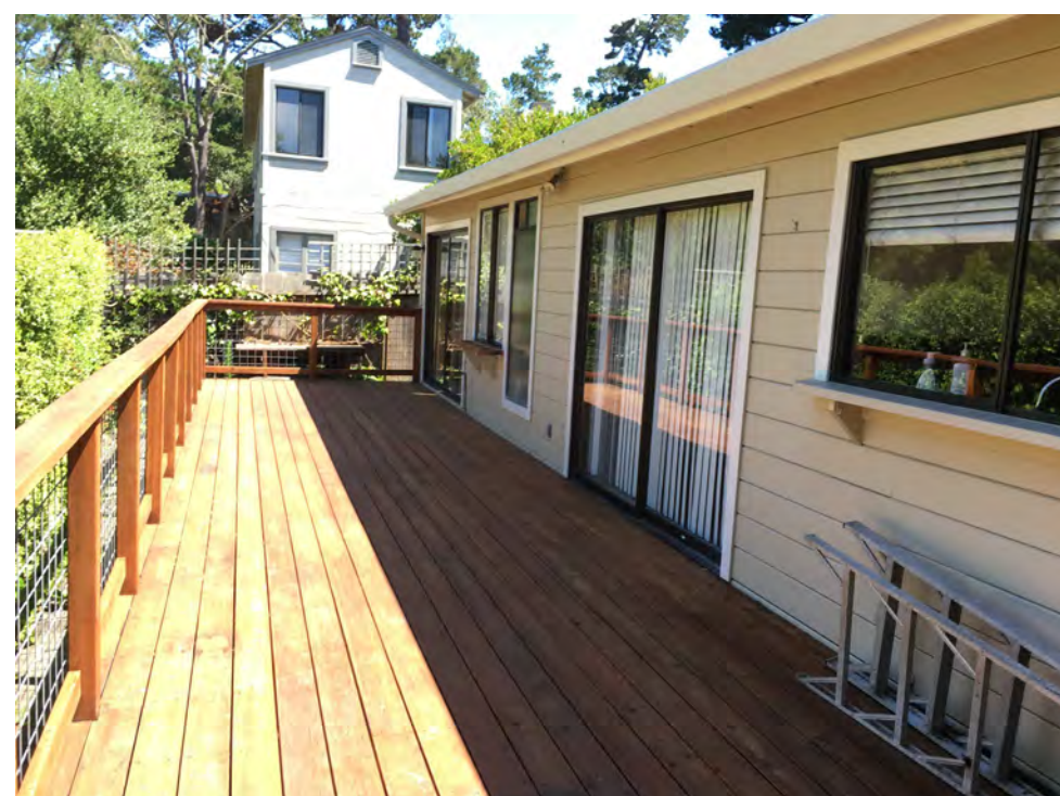
EXISTING DECK LOOKING NORTH
