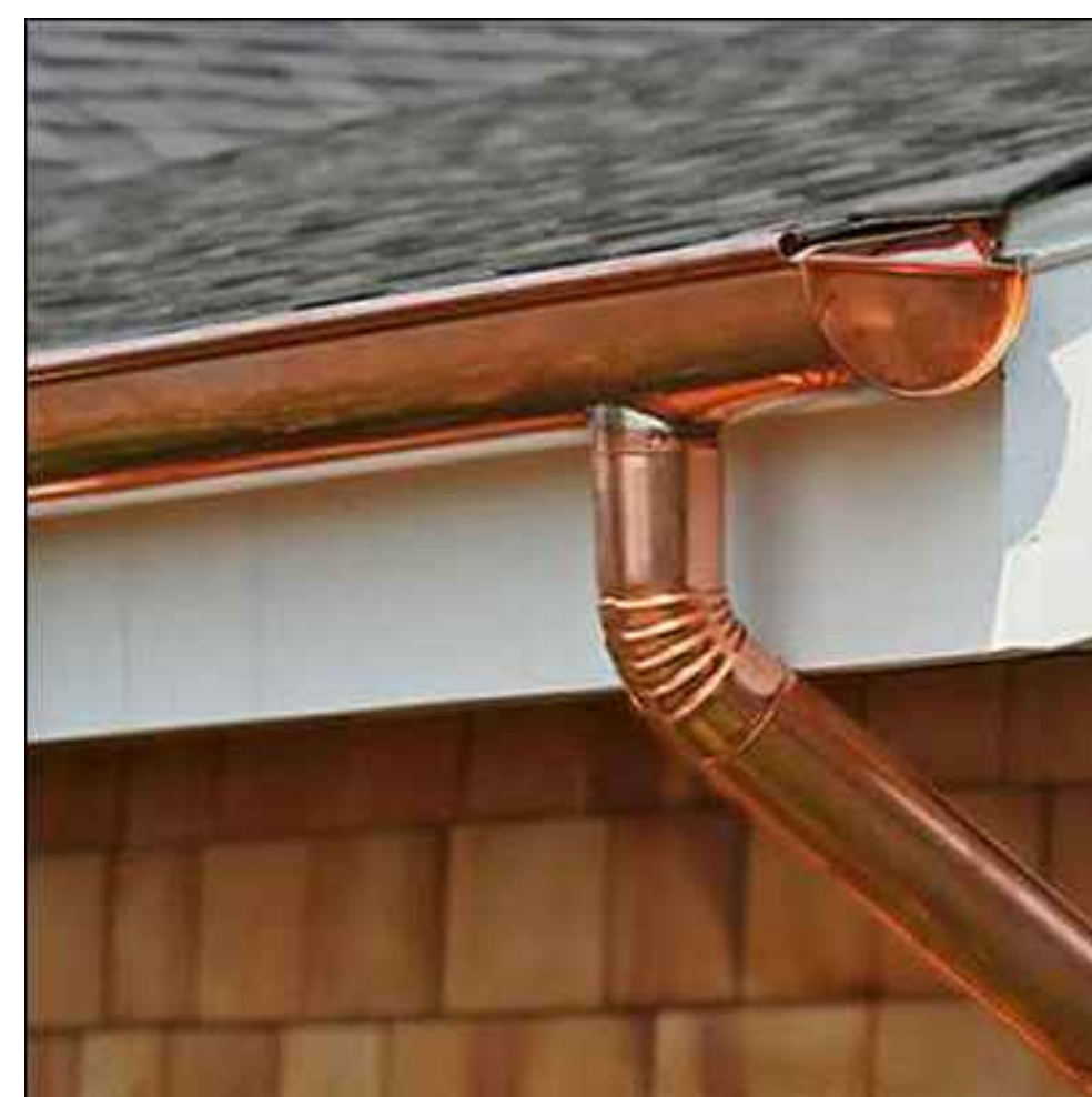
7 COPPER GUTTERS AND DOWNSPOUTS
