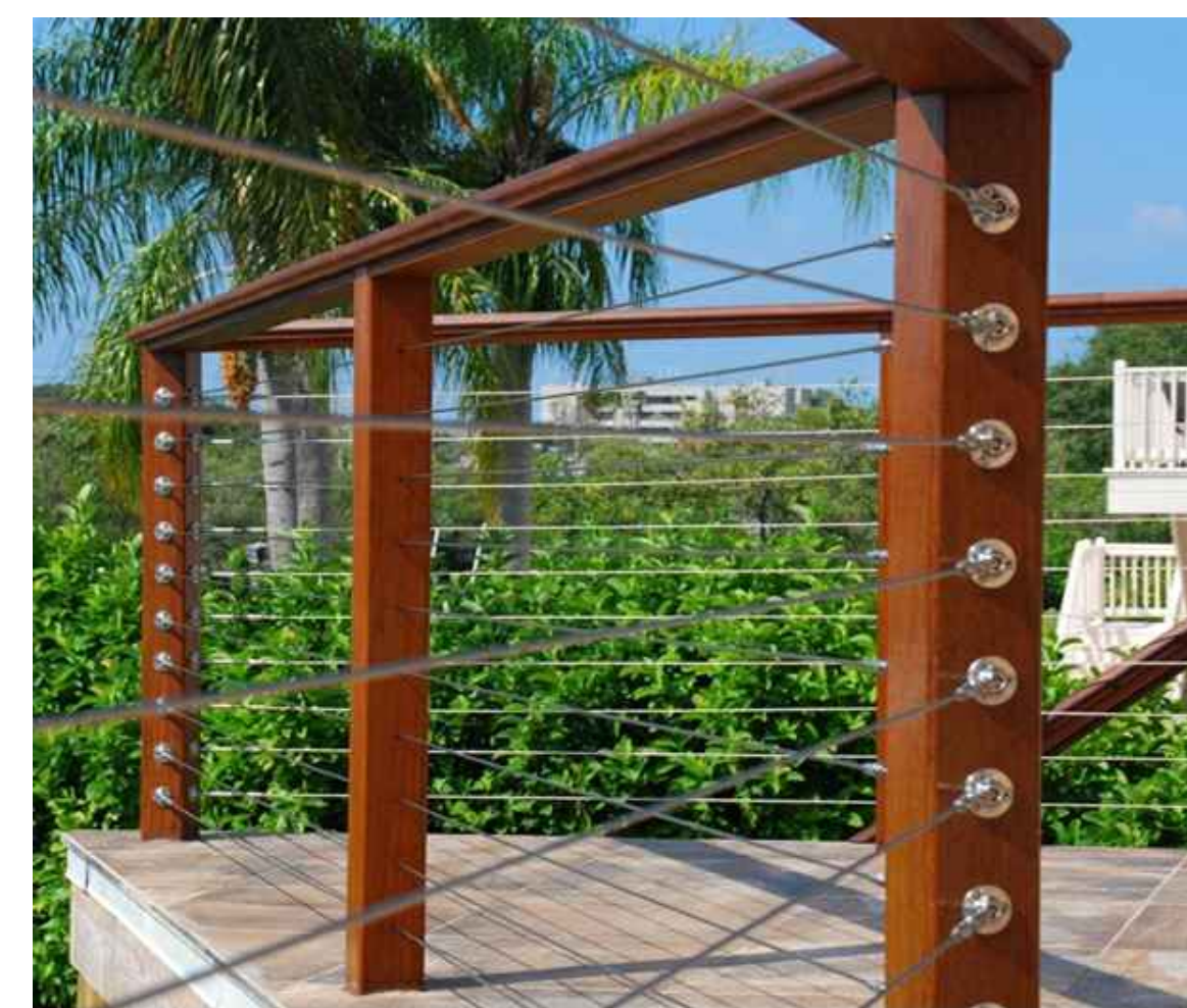
8 CABLE RAILING W/ REDWOOD TOP RAIL
