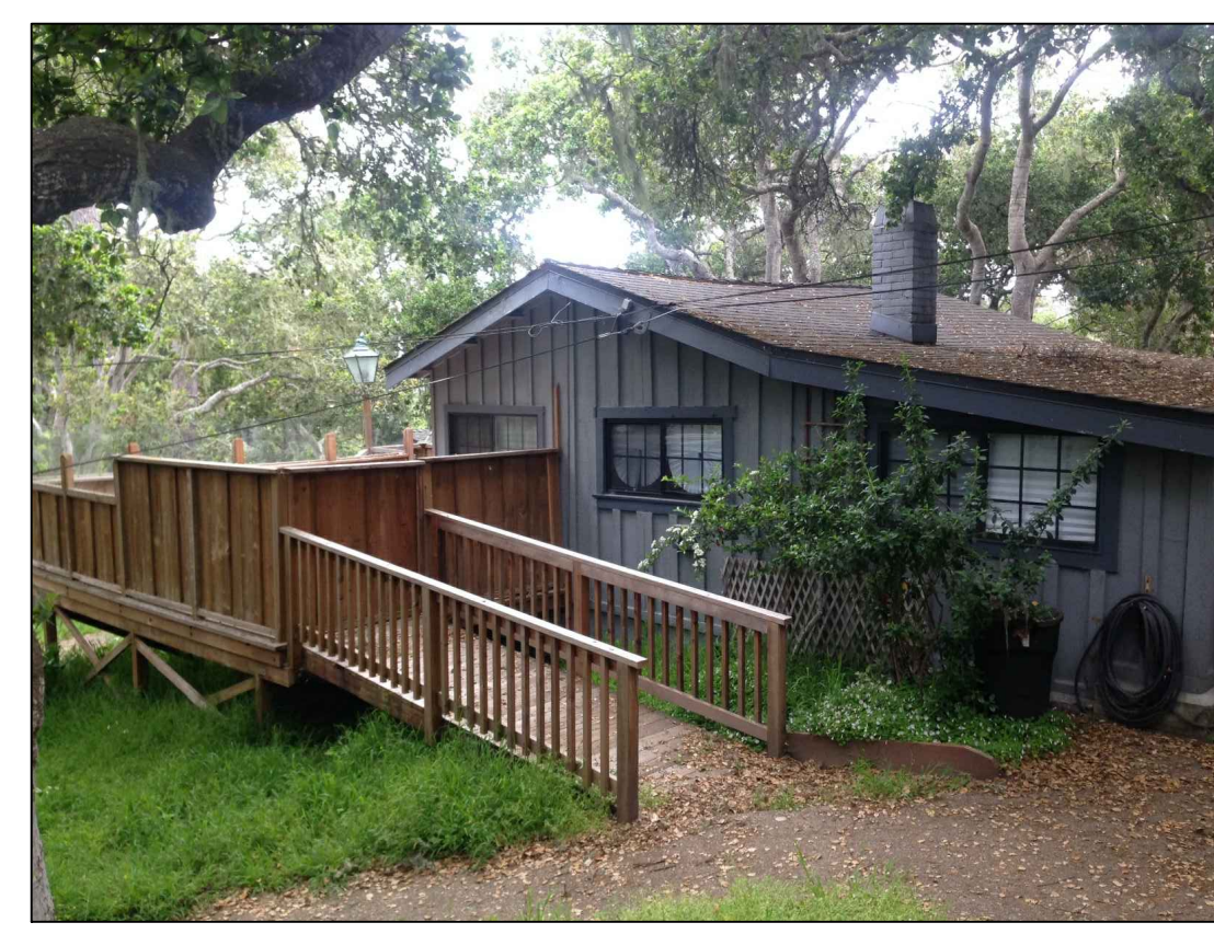
"The Cabin" view from south, present
