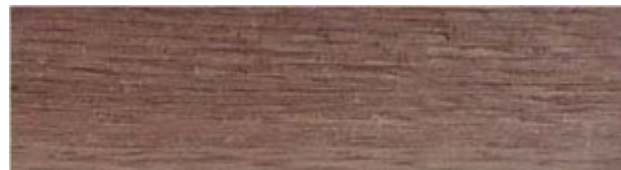
CEDAR RAFTER TAILS & GARAGE DOOR STAINED
