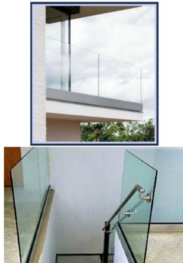
12 FRAMELESS GLASS GUARDRAIL & STAINLESS STEEL HANDRAIL
