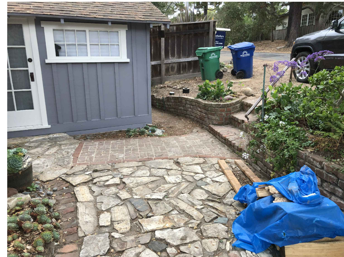
FRONT STONE & BRICK PATIO & BRICK WALLS TO REPLACE
