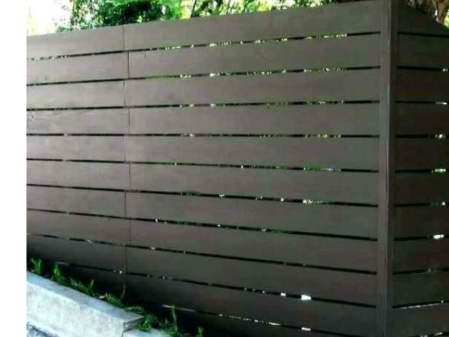
SIDE YARD FENCE - SPACED HORIZONTAL WOOD BOARDS, FENCE WILL SLOPE TO MATCH SITE SLOPE
