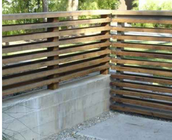
FRONT YARD SPACED WOOD FENCING & BOARD FORMED CONC. WALLS
