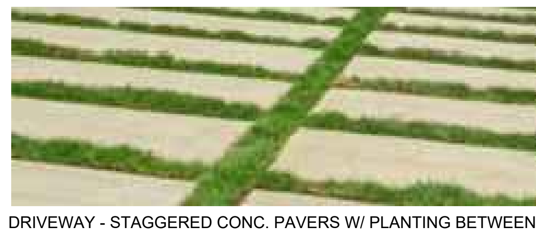
DRIVEWAY - STAGGERED CONC. PAVERS W/ PLANTING BETWEEN
