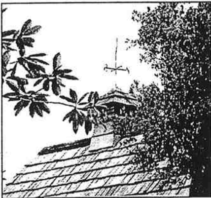
Architectural details contribute to character of the building and their use is encouraged.
