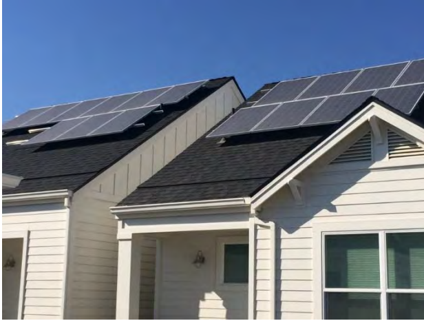
Photo: Rooftop solar panels at the 2500 R Street Community Development. Sunverge Energy https://cdn.leanegroup.org/wp-content/uploads/2500R-solar-on-roof-900x675.jpeg
