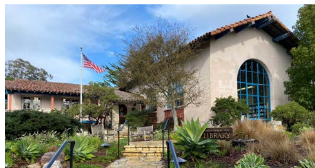
Architectural Figure 1: Existing Library - Exterior
