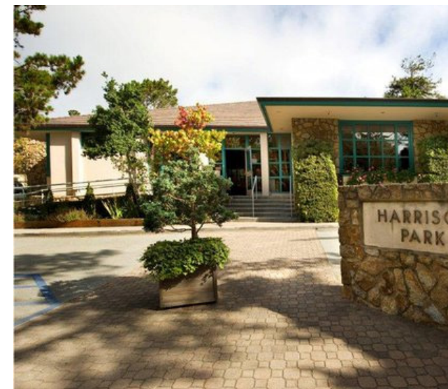
Architectural Figure 3: Existing Library - Exterior
