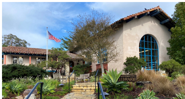
Architectural Figure 1: Existing Library - Exterior
