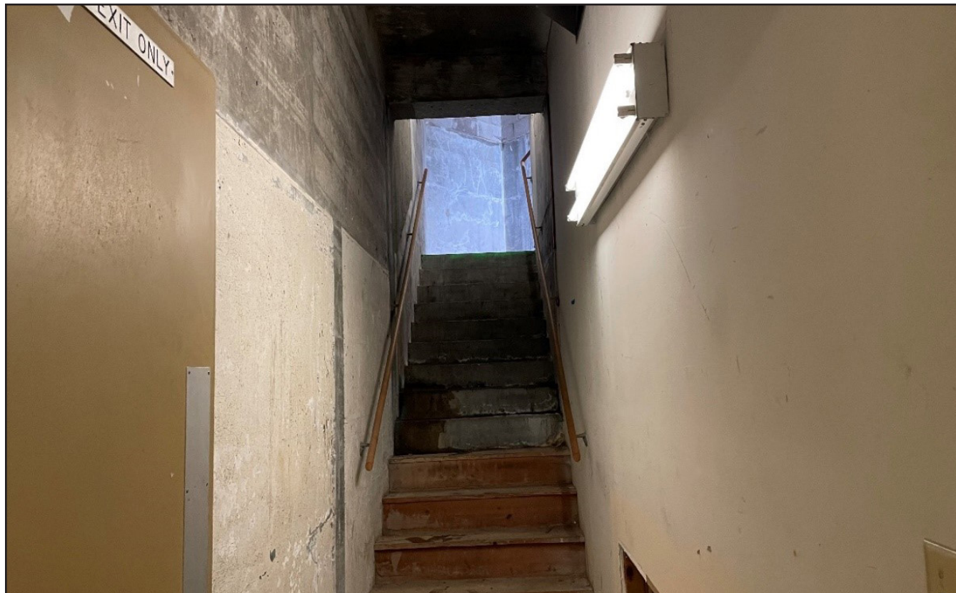
Structural Figure 8: Basement Entrance
