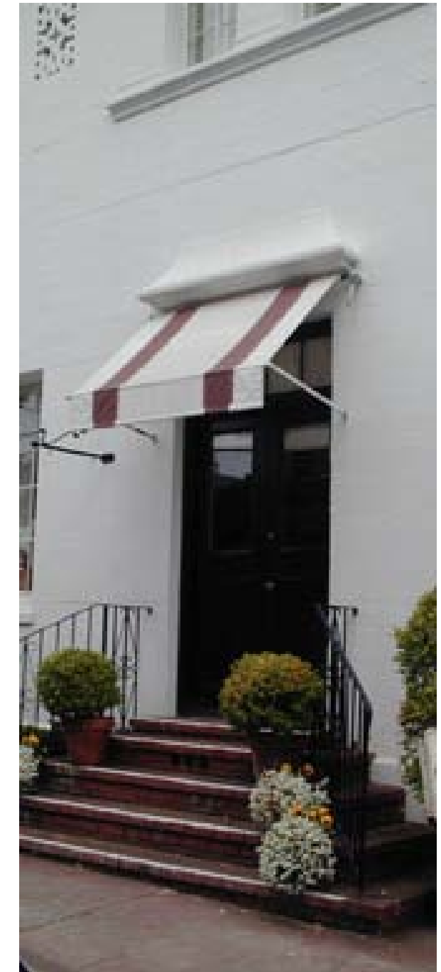
AWNINGS FIT IN OPENING WITH VALANCE
