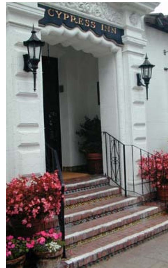
DECORATIVE STAIRS AND RAILINGS
