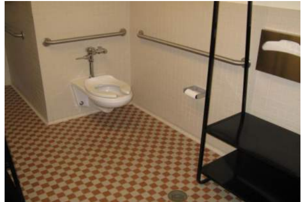
M2. South Portion - Chorus Level Men's Restroom and Dressing Room
