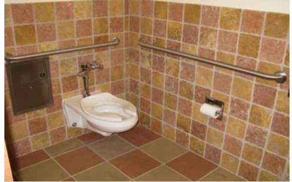
R2. South Portion - Conductor's Level Women's Restroom
