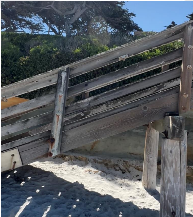
Figure 4: Stair 4 Guardrail Post/Split Stringer from Landing to Bottom of Stairway
