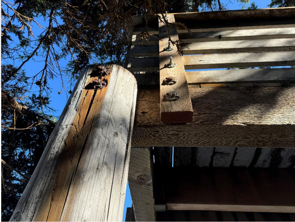
Figure 10: Post to Landing Bolted Connection
