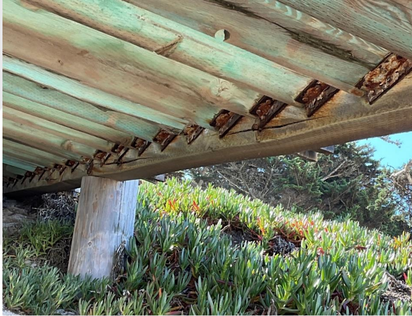
Figure 5: Stair 4 Stringer from Top of Stairway Upper Landing
