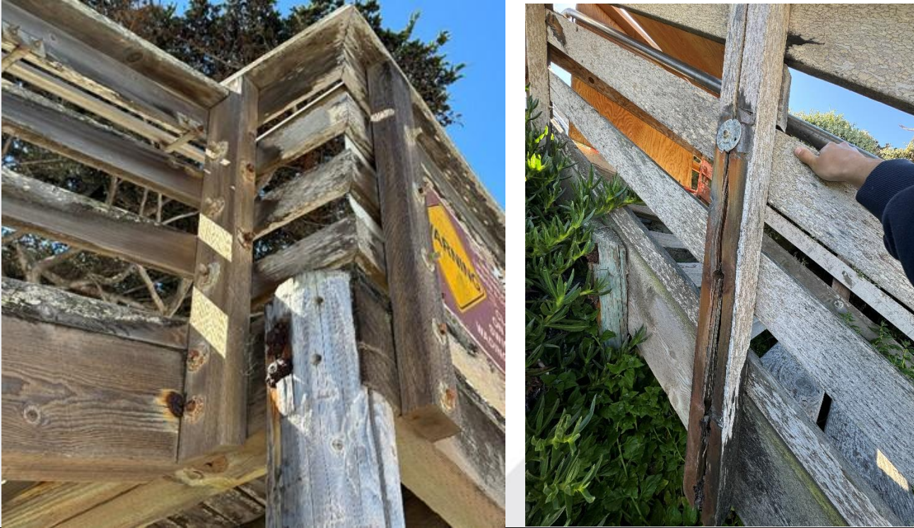
Figure 7: Post to Landing Bolted Connection
