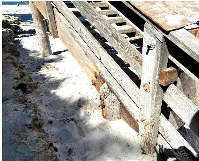
Figure 4: Stair 4 Guardrail Post/Split Stringer from Landing to Bottom of Stairway
