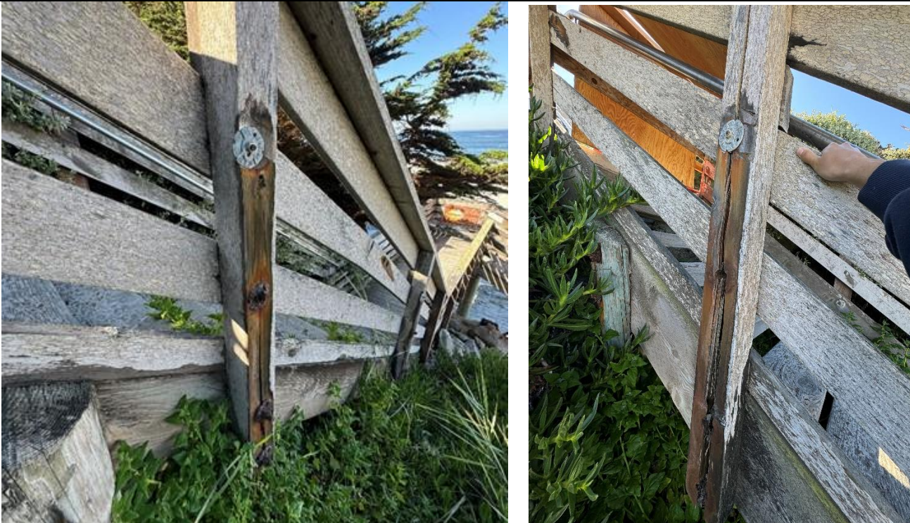
Figure 8: Guardrail Posts-Stringer Bolted Connection
