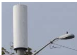
A Closer Look at 5G Equipment that is Being Instal...
