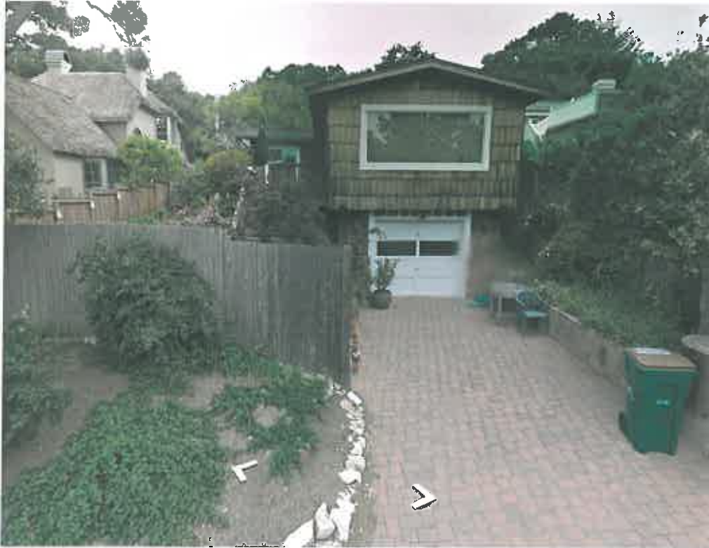
Project site – Facing north on Santa Lucia
