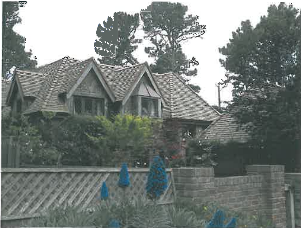
Adjacent Lot to west with similar style residence – Facing southwest on 2 nd Ave
