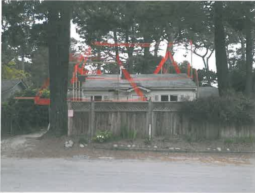
Front of project site – Facing south on 2 nd Ave
