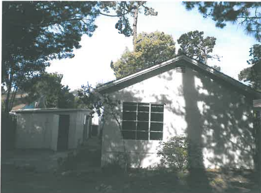
Rear of subject property
