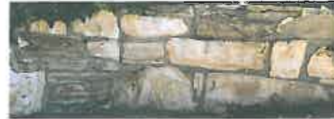
NEW STONE VENEER ON BASE OF HOUSE TO MATCH EXISTING STONE RETAINING WALL (PHOTO)
