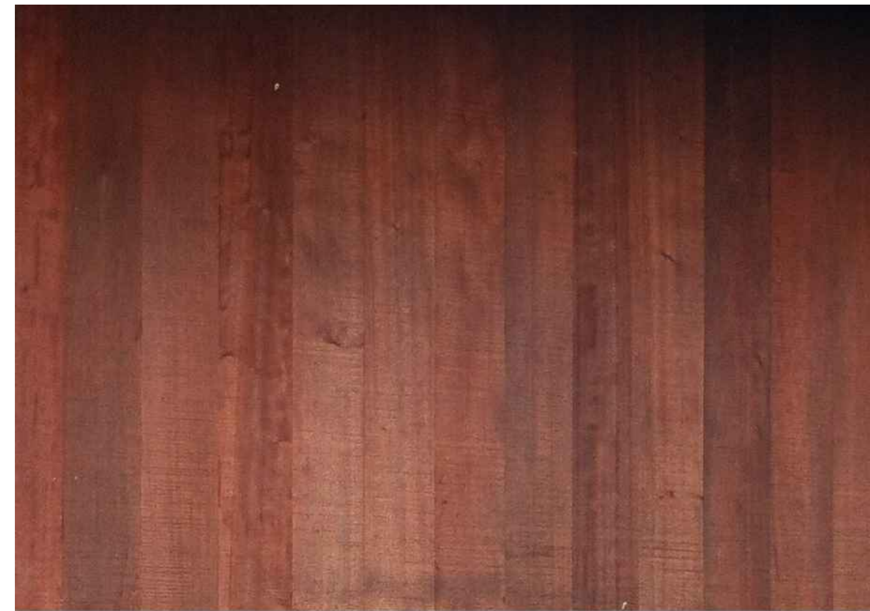
BUILDING EXTERIOR WALLS-EXISTING NATURAL PATINA REDWOOD SIDING
