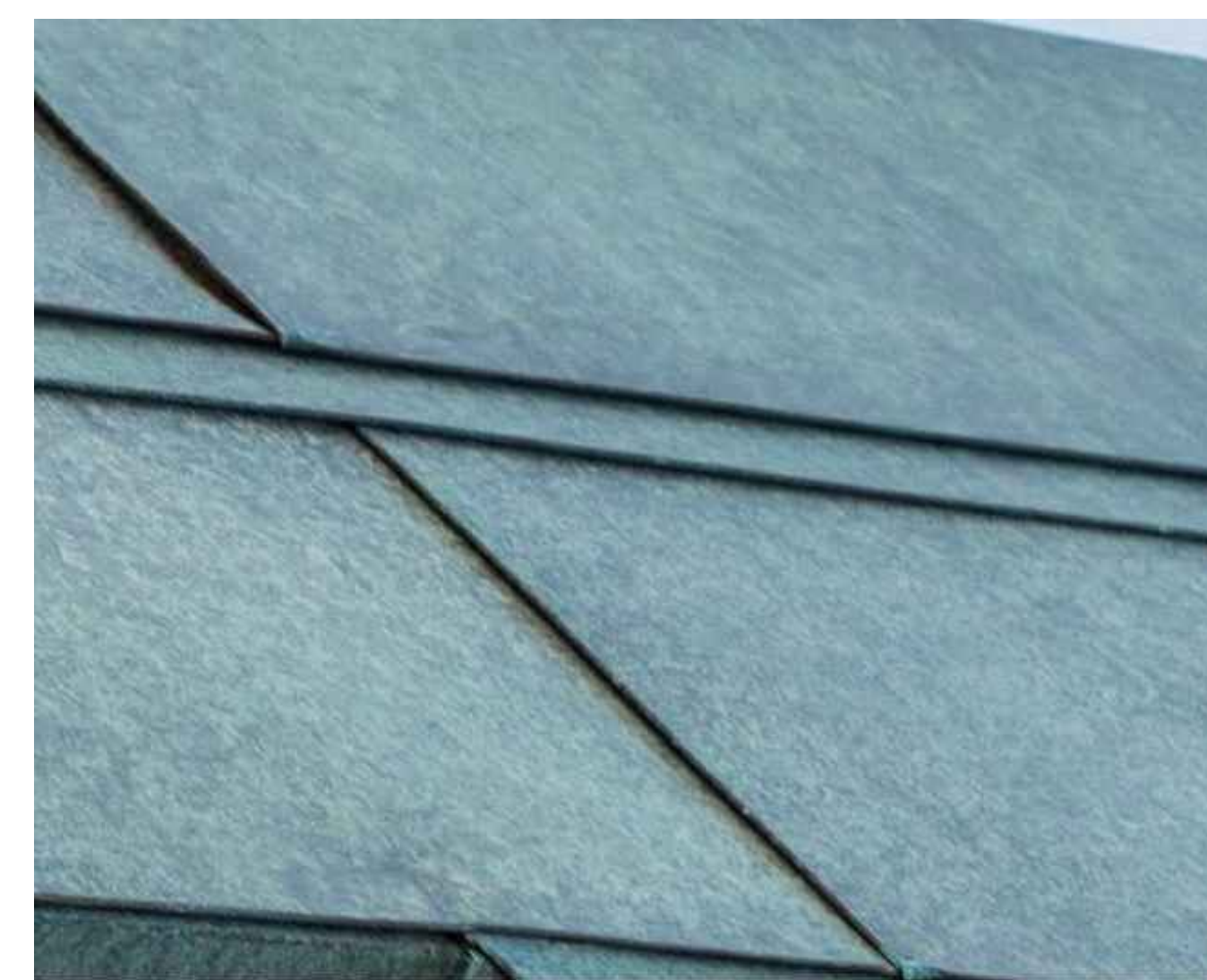
BUILDING ROOF-EXISTING WEATHERED COPPER
