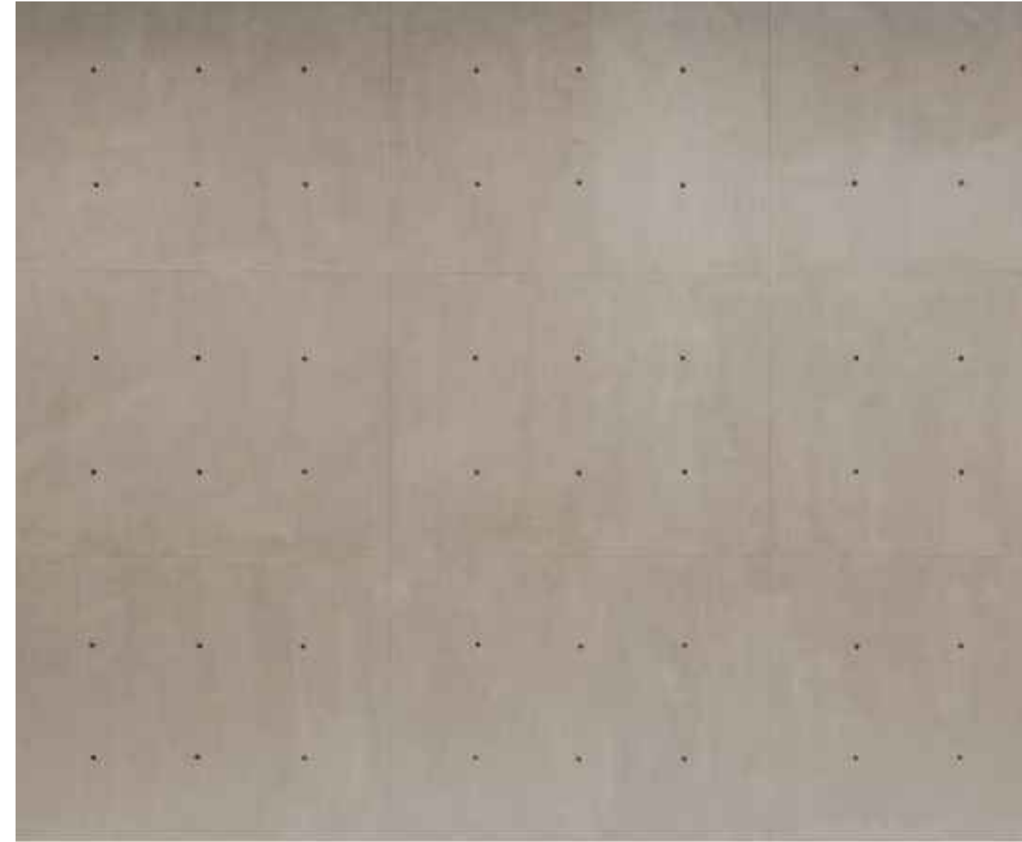
BUILDING EXTERIOR WALLS-NEW FORMED IN PLACE CONCRETE
