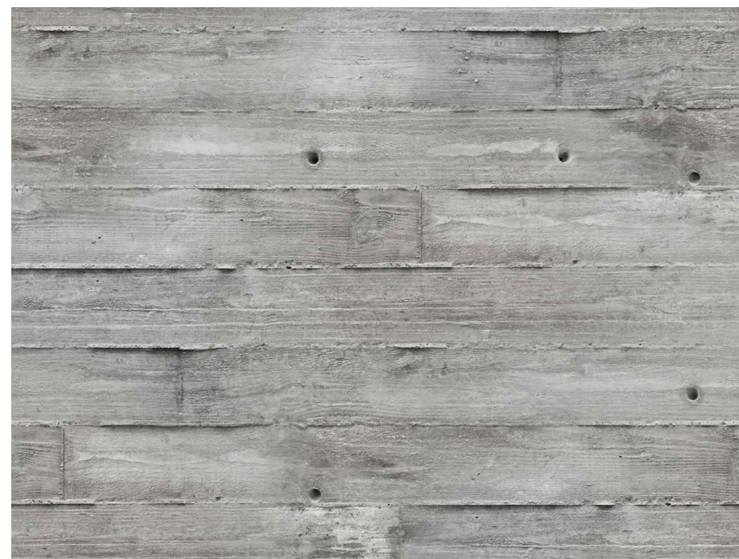
BUILDING EXTERIOR WALLS-NEW BOARD-FORMED CONCRETE
