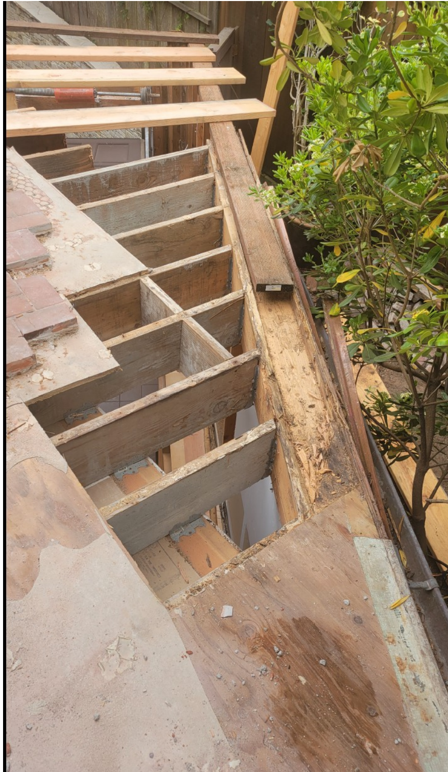
Photograph of rot damaged deck framing and wall framing to be replaced or repaired. The rotten guardrail along the wall line has been removed and hauled off. This view is standing on deck facing the street.
