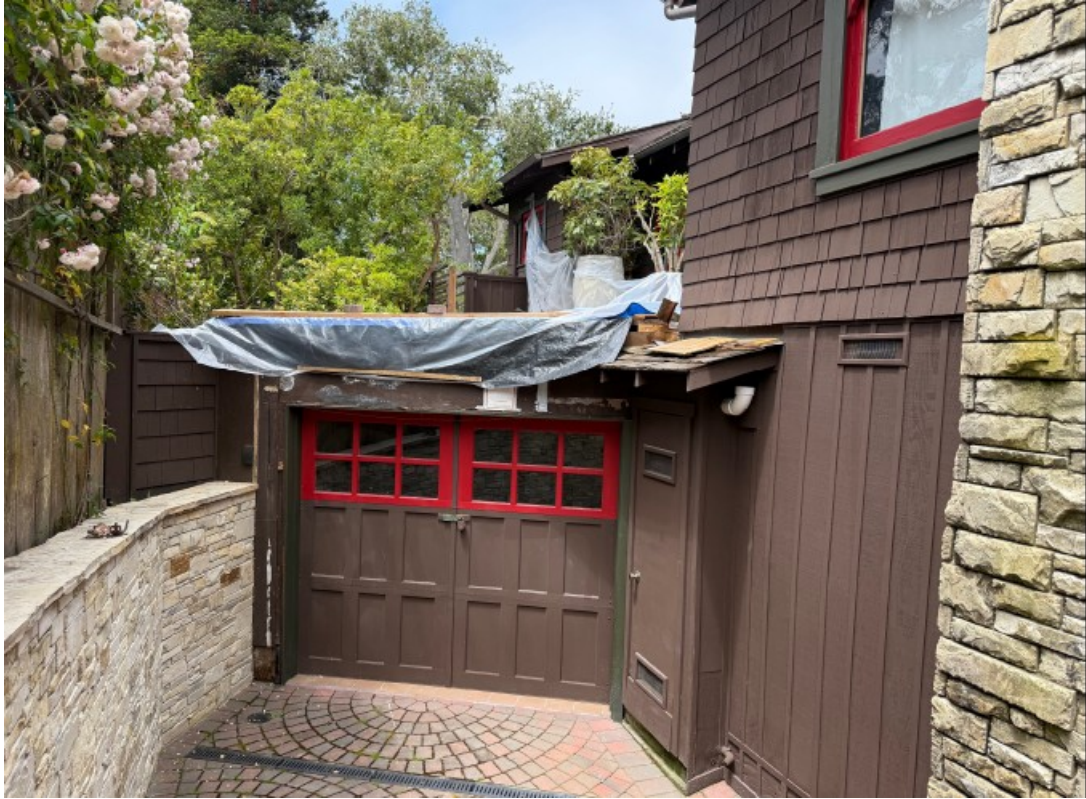
Front Elevation photograph of garage and damaged roof deck. Note: Guardrail has been removed and hauled off.
