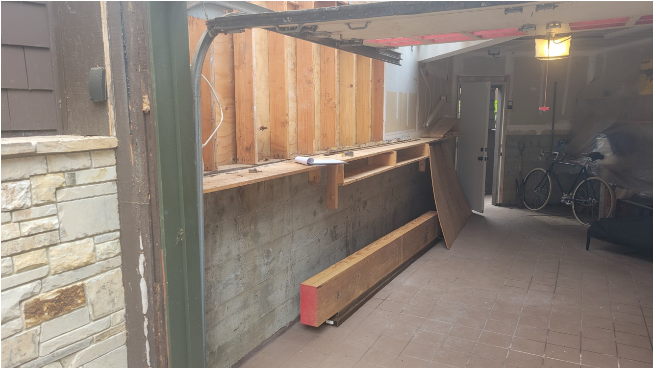
Photo of rot damaged wall. This photo was taken standing in driveway looking into the garage. The wall on the left is rotten with temporary plywood nailed to the outside. Sheetrock has been removed. The concrete retaining wall inside the garage on left will remain in place.
