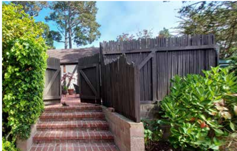
EXISTING GATE & FENCE CONDITIONS
