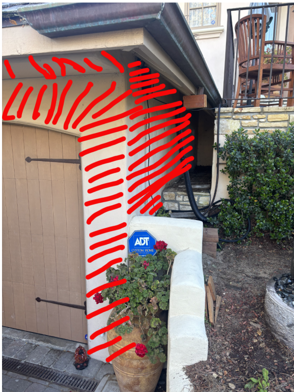
Proposed Montgomery Gold stone veneer to match existing chimney veneer
