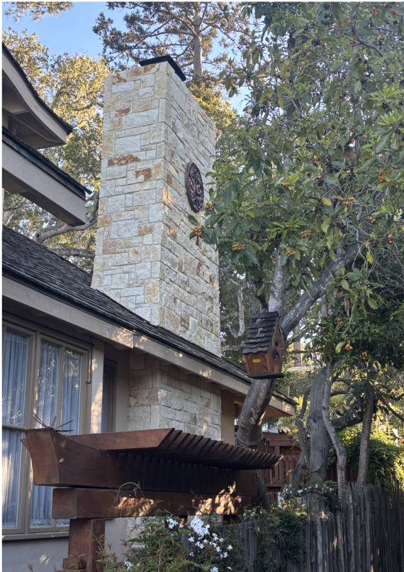
Proposed Montgomery Gold stone veneer to match existing chimney veneer
