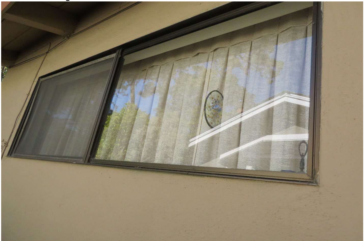
Window #7 - dining room
