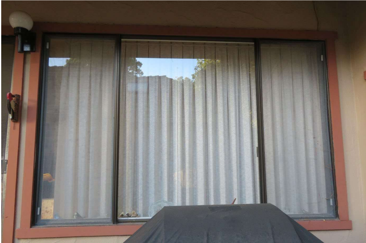
Window #2 - living room
