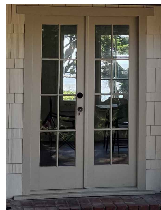
WOOD DOORS MATCH EXISTING WITH TRUE-DIVIDED LIGHTS
