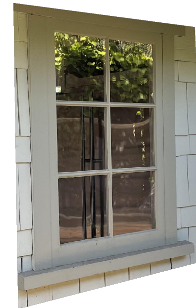
WOOD WINDOWS MATCH EXISTING WITH TRUE-DIVIDED LIGHTS
