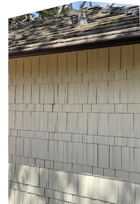
EXISTING WOOD SHINGLES / ROOF SHAKES
