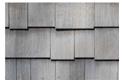
NEW WOOD SHINGLES AT NEW ADDITION
