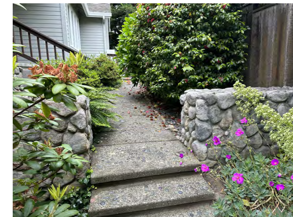
EXISTING WALK TO FRONT DOOR
