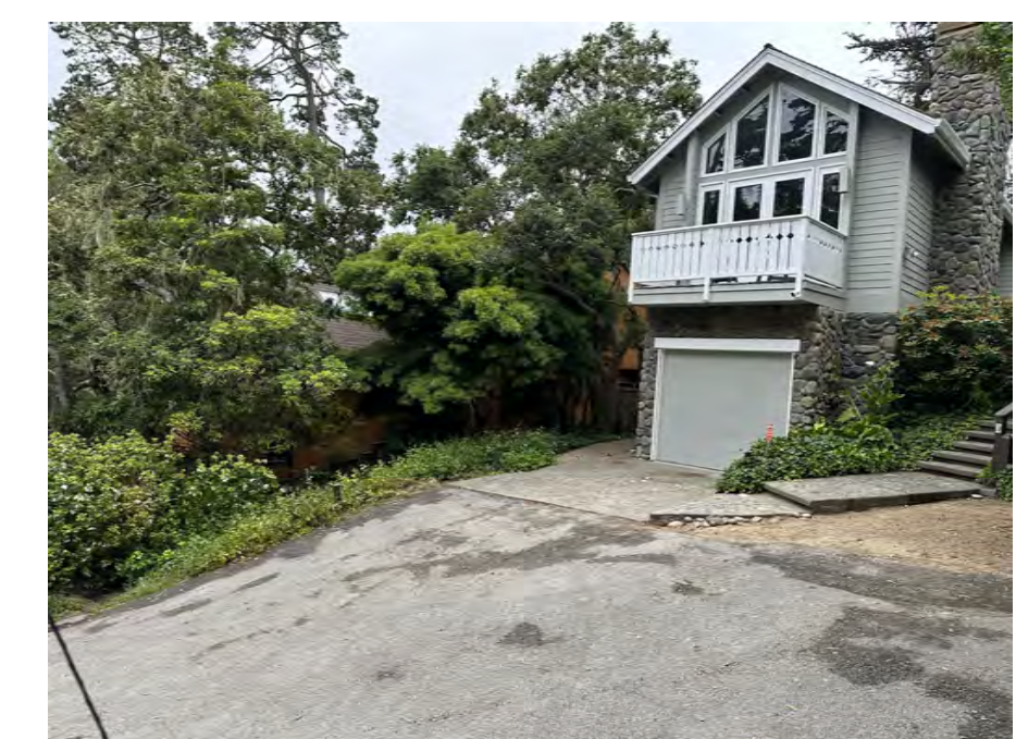
FRONT CONCRETE DRIVEWAY
