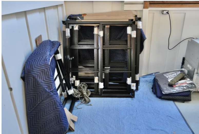
Figure 4. Image of restored and repainted steel windows.
