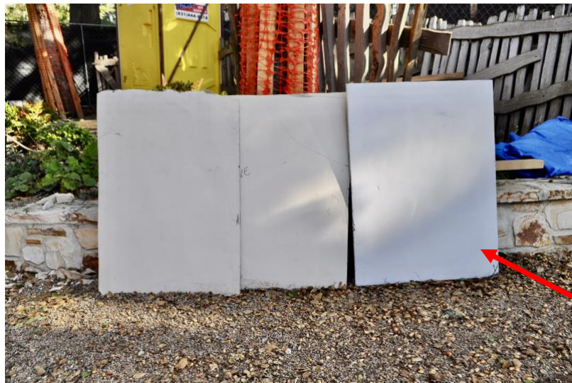
Figure 3. Image of original stucco wall section (far left) and the proposed mock-up (far right).
