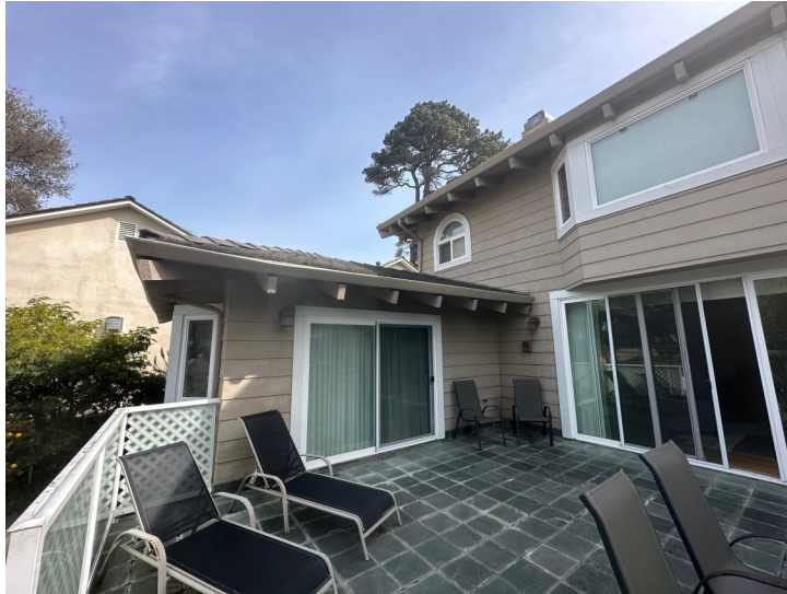
Lower Deck with Lattice and Glass Railing
