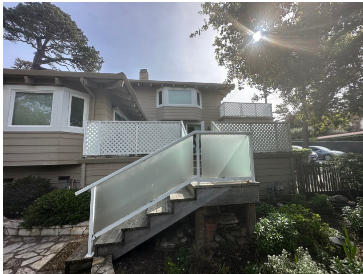
Lower Deck with Lattice and Glass Railing and Stair No Lattice Glass Railing
