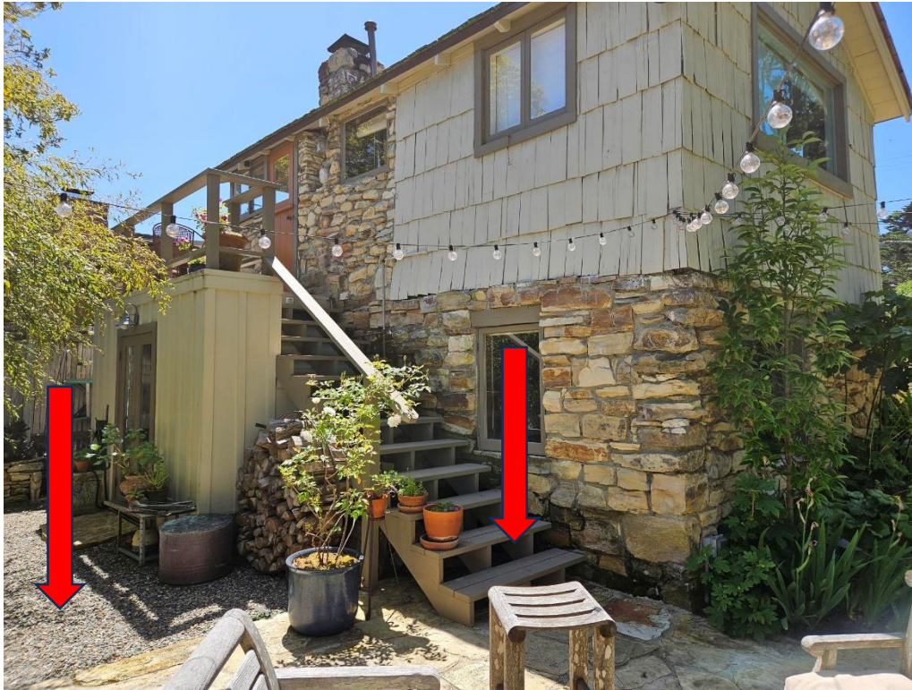
Figure 3: Arrows indicate the location of the ADU and the non-historic stairs.
