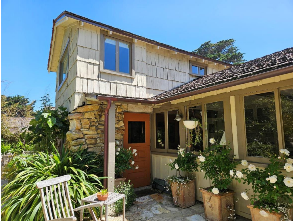
Figure 4: View of original 1921 servant's quarters and 1927 two-story addition.
