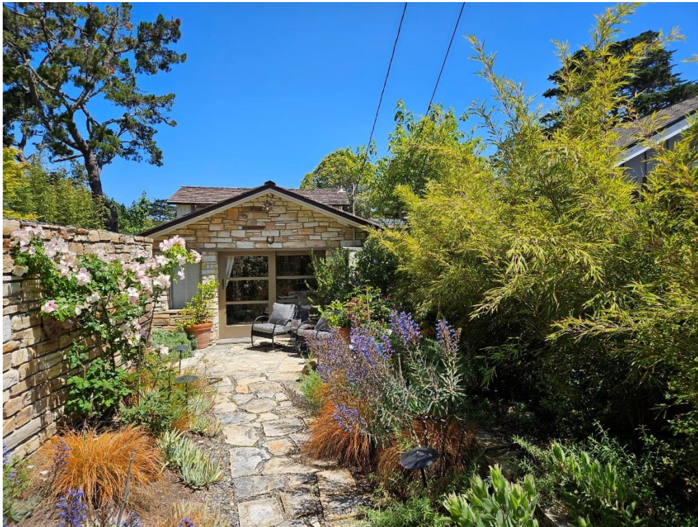
Figure 1: View of front elevation.
