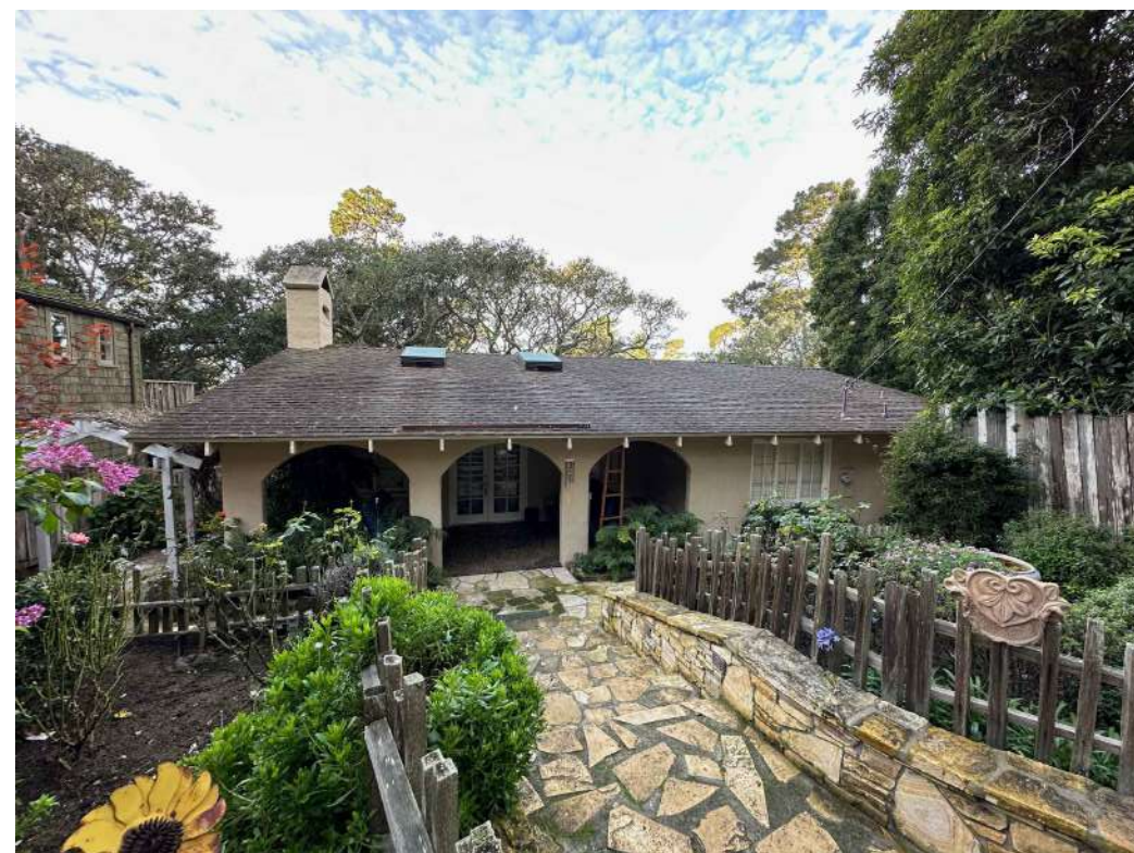
FRONT OF HOUSE LOOKING WEST
