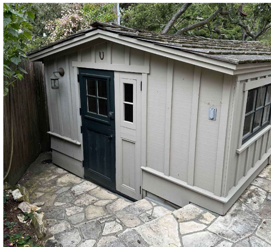
REAR ELEVATION OF GARAGE
