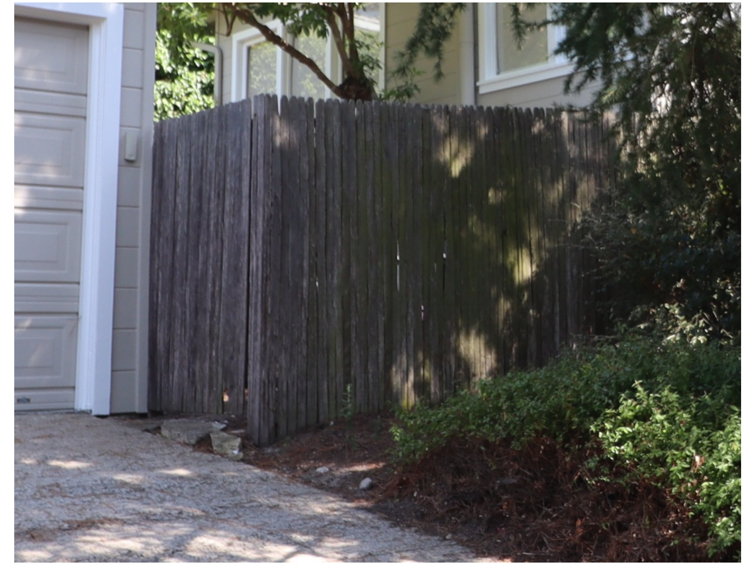
EXISTING SPLIT PALING WOOD FENCE (72" TALL MAX)
