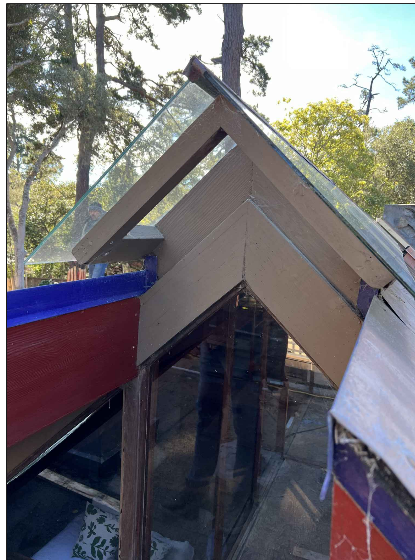
A EXISTING GABLE RIDGE FASCIA PHOTO NTS
