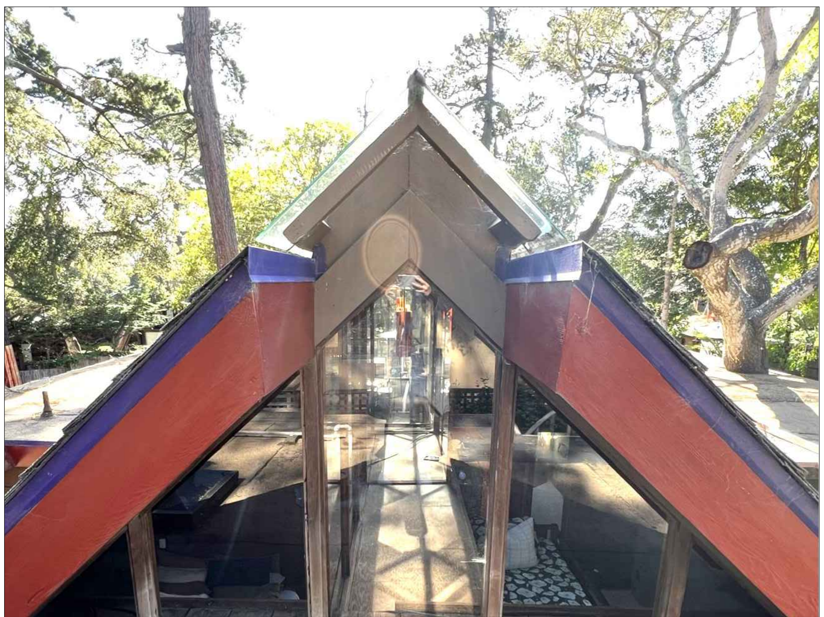
C EXISTING RIDGE SKYLIGHT PHOTO NTS
