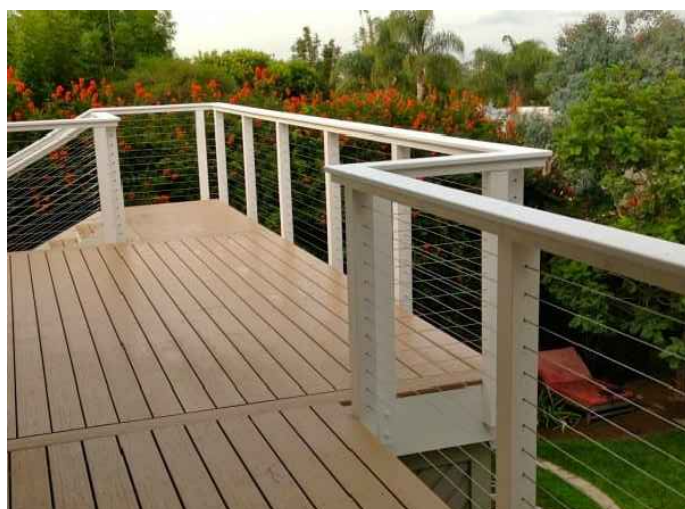
PAINTED REDWOOD DECK, PAINTED WOOD GUARDRAIL W/ ALUM. CABLING BETWEEN POSTS
