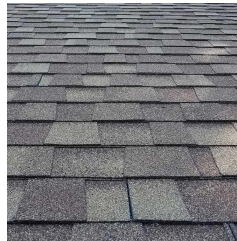
New Roof (Under separate, approved permit)
