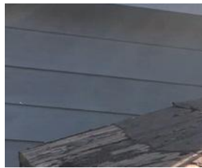
“New” (Existing) Siding
