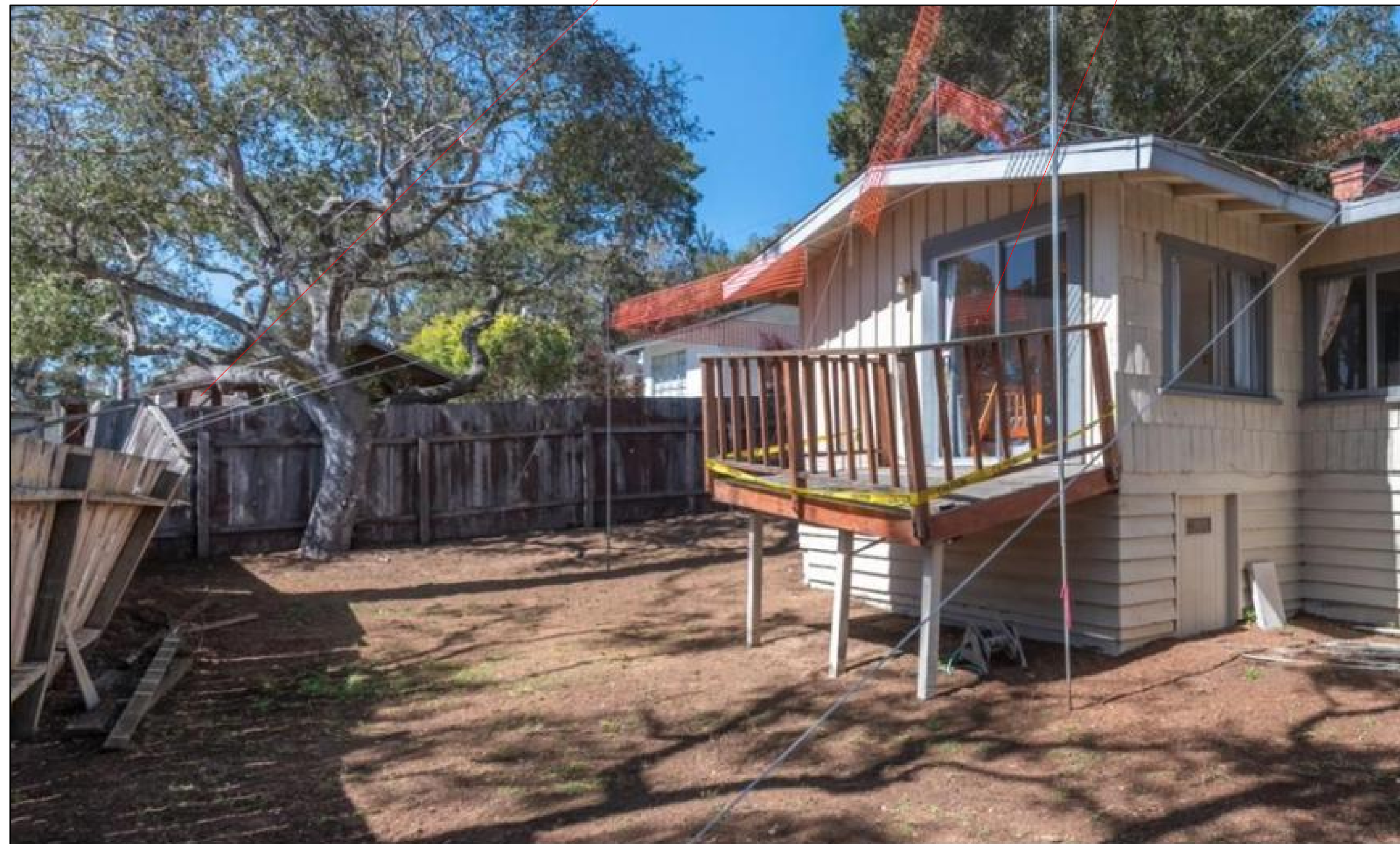
Existing Conditions at southern fence & Deck #2
