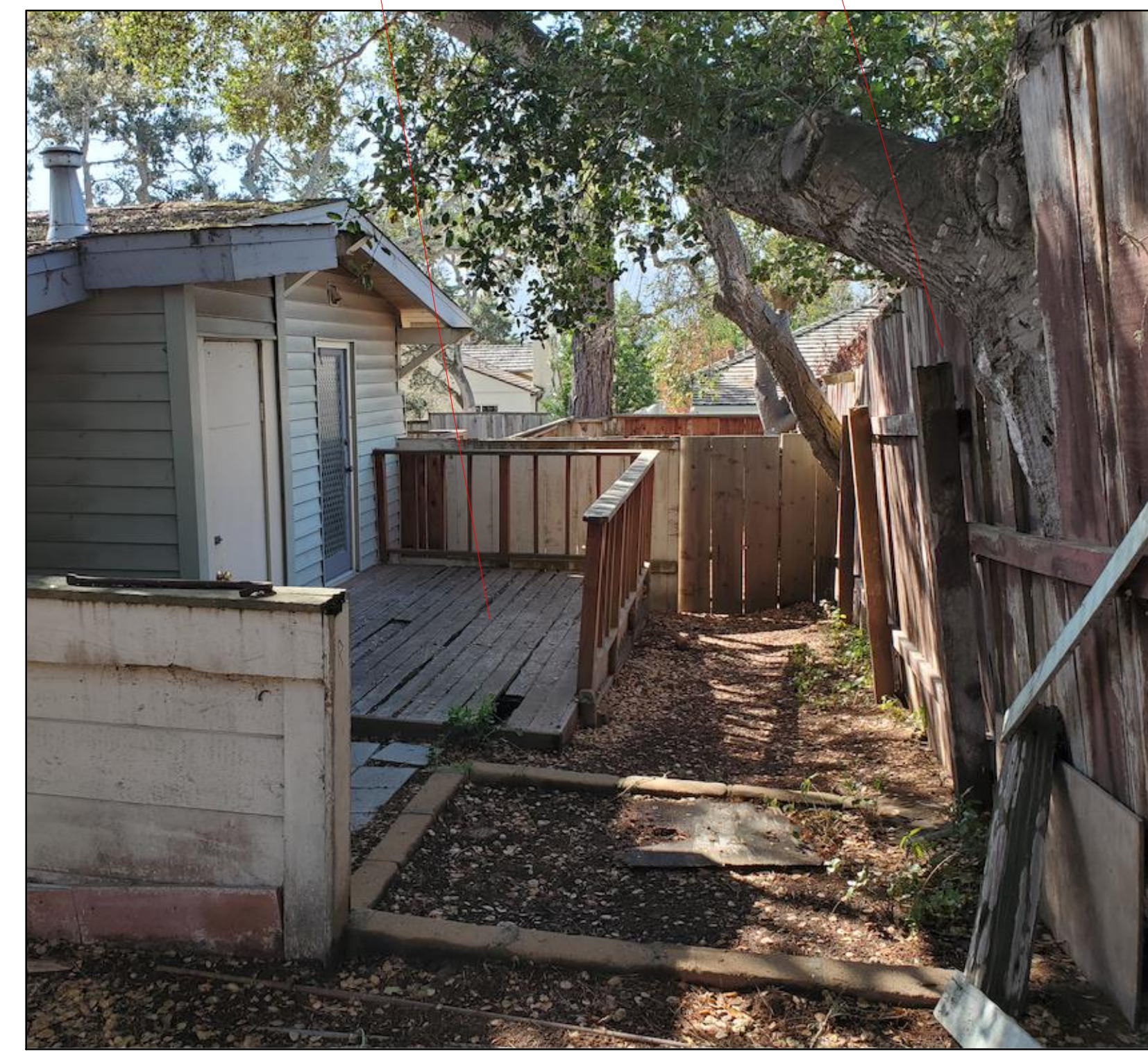
Existing Conditions at western fence & Deck #4
