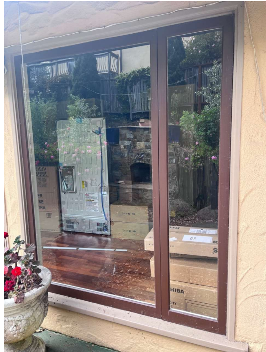
10. Living Room Window (Right Side of Slider)
