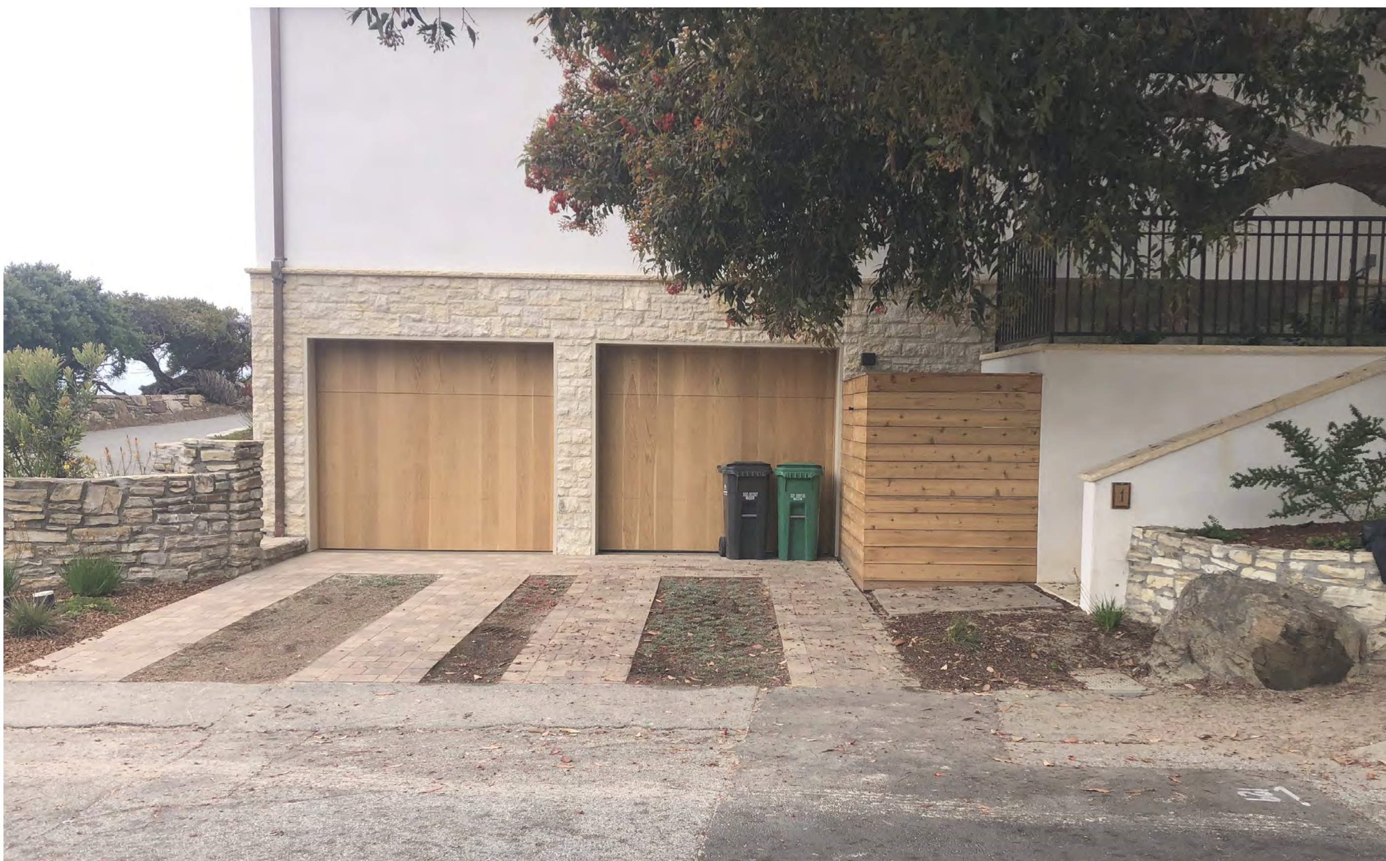
3 SITE PHOTO: EXISTING DRIVEWAY
