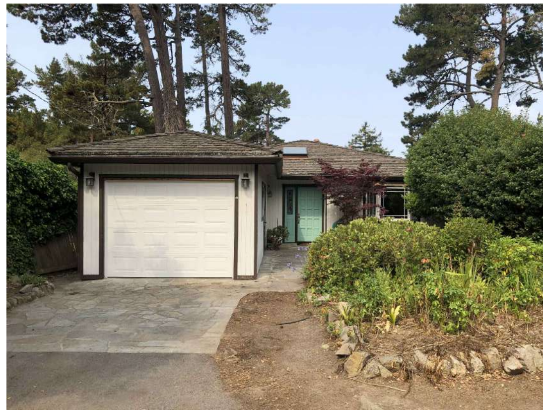
FRONT OF (E) HOUSE LOOKING WEST.
