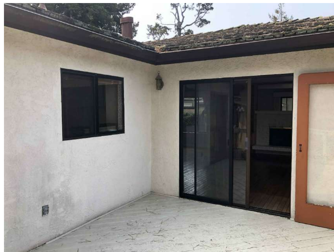
REAR DECK LOOKING SOUTHEAST.
