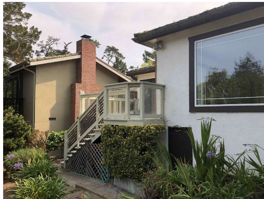
REAR OF (E) HOUSE LOOKING NORTHEAST.
