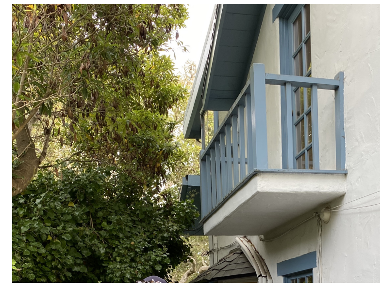
DEMO JULIET BALCONY ON NORTH FACADE
