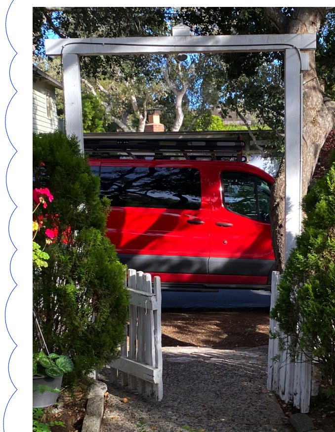
(E) ARBOR AT FRONT (EAST) GATE. REPLACE WITH SAME STYLE, BUT NATURAL WOOD TO MATCH NEW GRAPESTAKE FENCING. MAXIMUM HEIGHT 7'.
